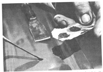
(4) Work this mixture of gel coat, fibers and catalyst into the damaged area, using the sharp point of a putty knife or knife blade to press it into the bottom of the hole and to puncture any air bubble which may occur. Fill the scratch or hole above the surrounding undamaged area about 1/16".
