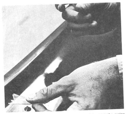
Lay a piece of cellophane over the patch to start the curing process. Repeat step 6, trimming patch when partially cured.
